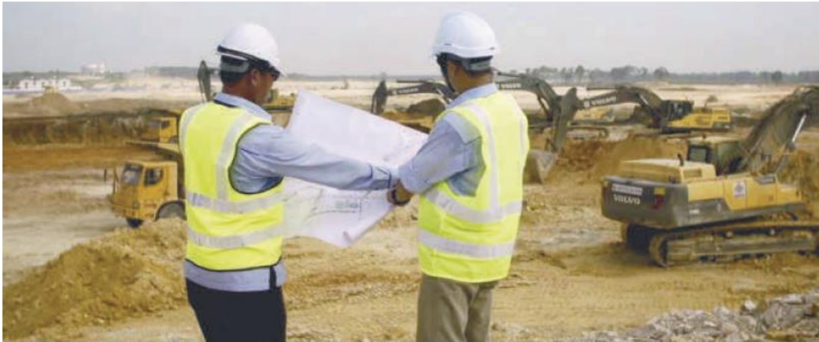
Advancecon Infra has more than 25 years of experience in civil engineering and infrastructure works. – ADVANCECON WEBSITE PIX
