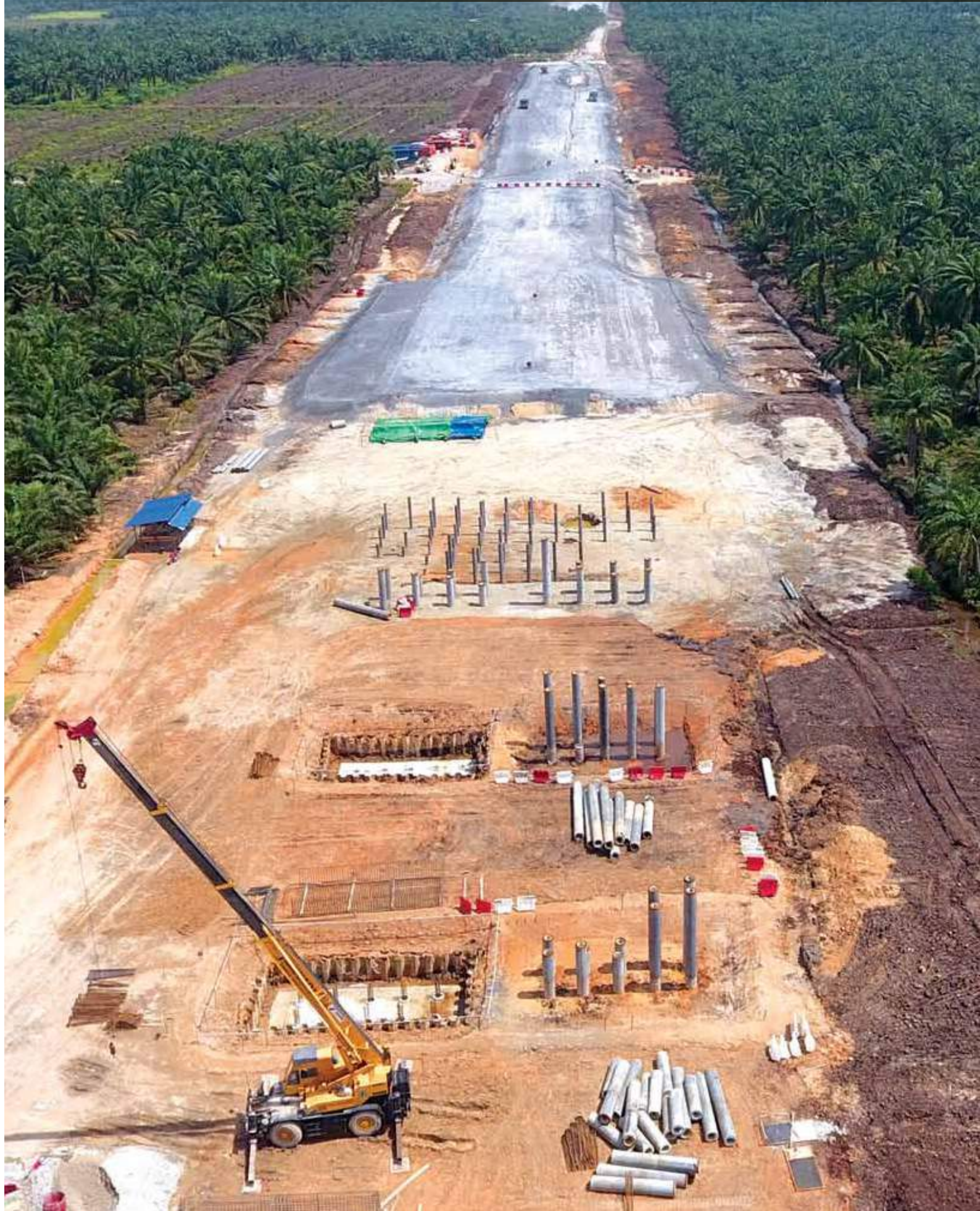
CONSTRUCTION AND COMPLETION OF CIVIL WORKS FOR WEST COAST EXPRESSWAY (FROM SECTION 1 - BANTING INTERCHANGE TO SOUTH KLANG VALLEY EXPRESSWAY)
