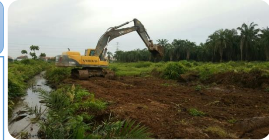
Clearing of project site
