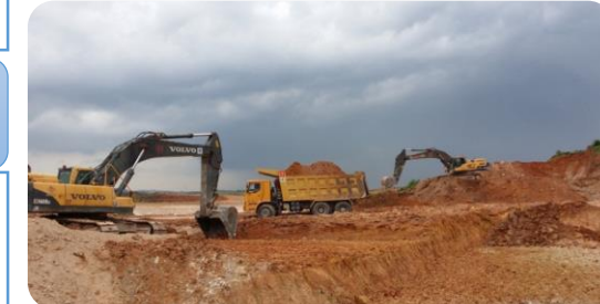
Hydraulic excavators loading soil
